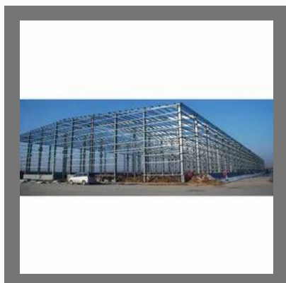
Pre Engineered Building Structure
