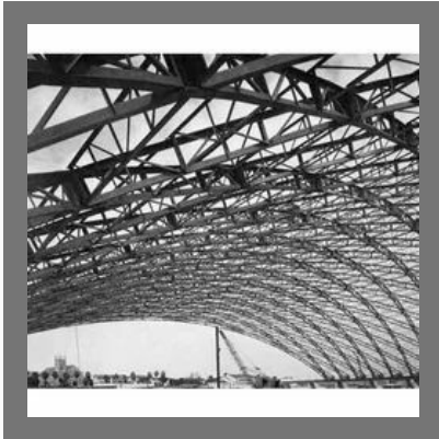
SS Roofing Structure
