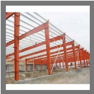
Building Roofing Structure
