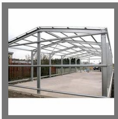
Mild Steel Pre Engineered Building Structure
