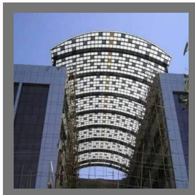
Residential Roofing Structure
