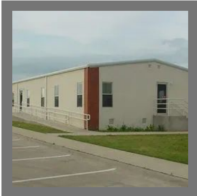
Prefabricated School Building
