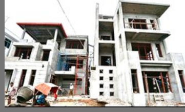
Civil Construction Work Contractors
