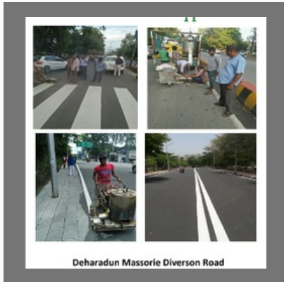
Road Marking Contractor
