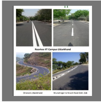
Road Marking Contractor
