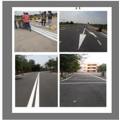
Road Marking Contractor
