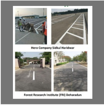
Road Marking Contractor
