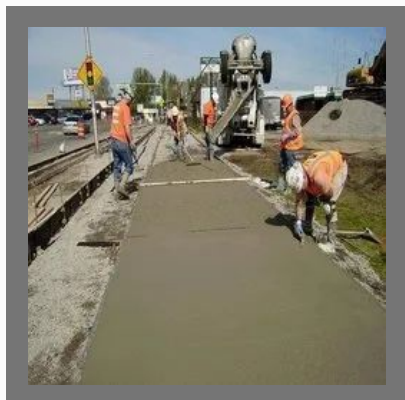
RCC Road Construction Services
