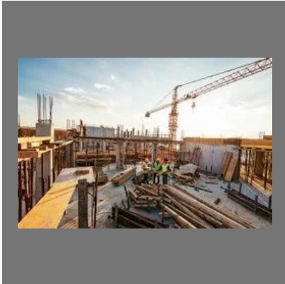
Building Construction Services
