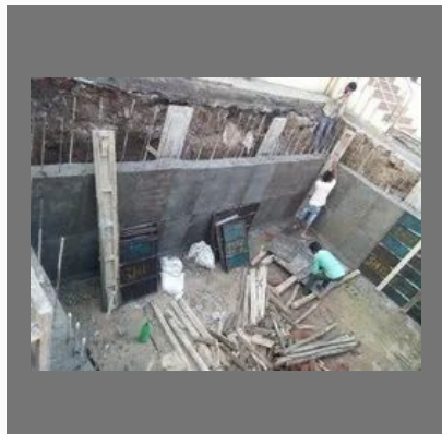
Water Tank Construction Services
