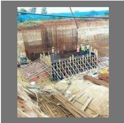
Building Construction Project
