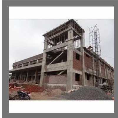
School Building Construction Services
