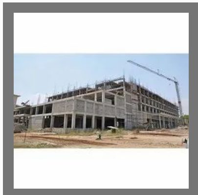
Industrial Construction Services
