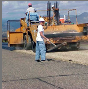
Road Construction Services
