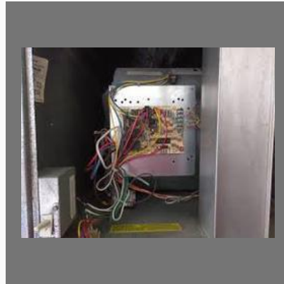
Air Cooler Repair Services
