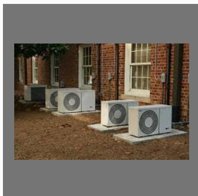
AC Repairing Services
