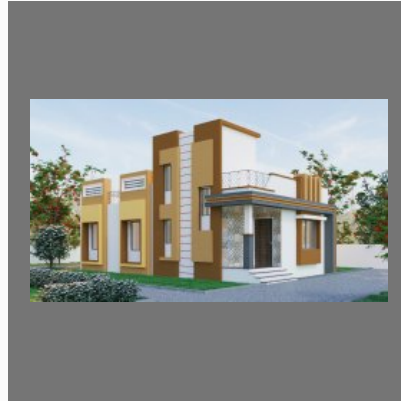
Building Construction Work
