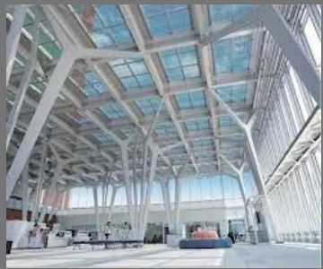
High Rise Structures Building Construction
