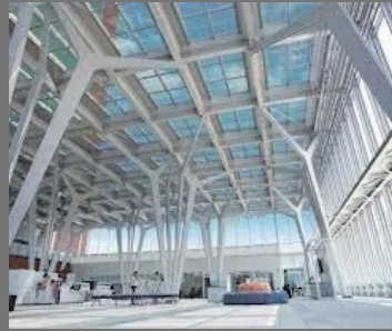
Public Sector Building Construction
