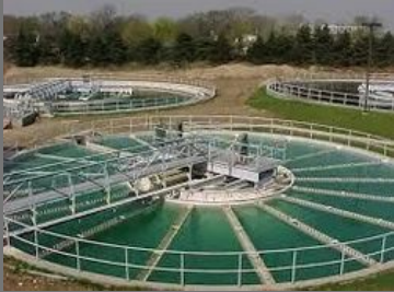
Water Treatment Plants
