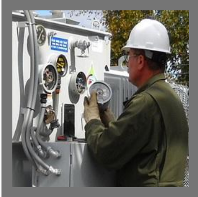
Power Transformer Repairing Service
