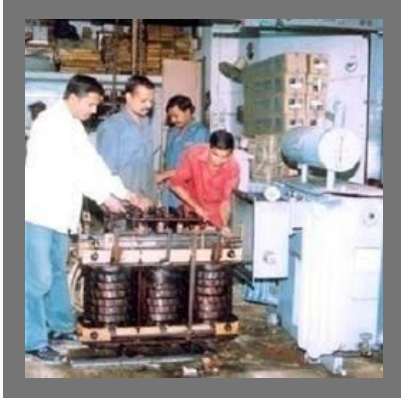
Control Transformer Repairing Service
