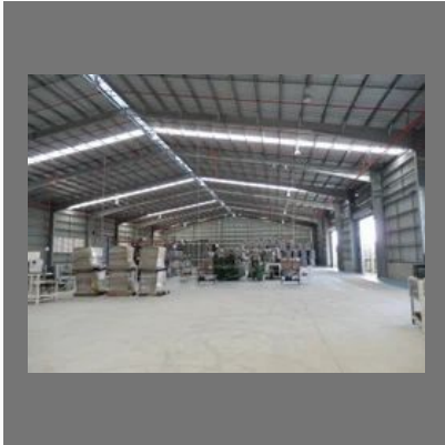
Mild Steel Structure Fabrication Shed
