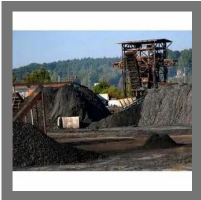
Coal Handling Services
