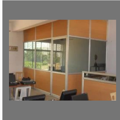
Aluminium Partition Works
