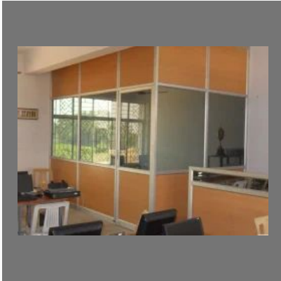
Aluminium Partition Works
