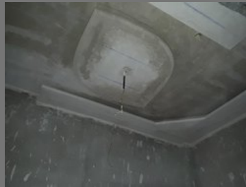
Gypsum Board Decoration Service For Home
