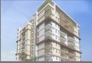
Commercial Construction Service
