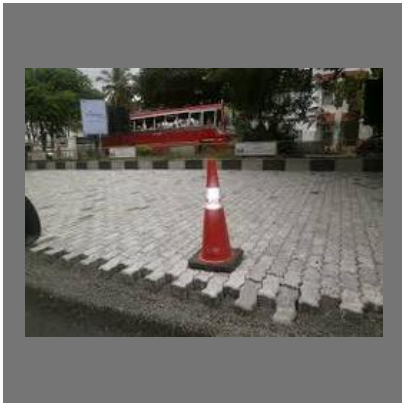
Interlocking Roads Construction
