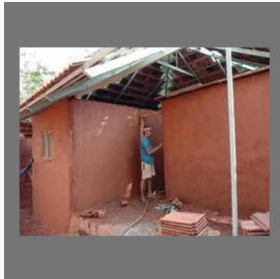
Mud House Construction Services
