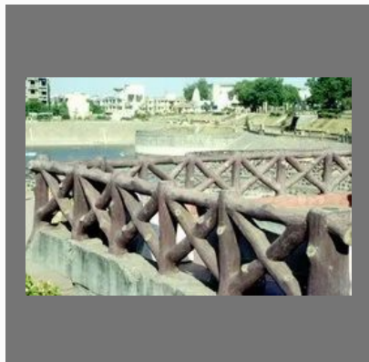
Artificial Tree Concrete Railing
