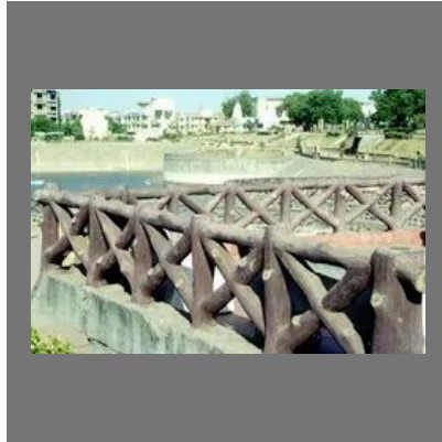
Artificial Tree Concrete Railing
