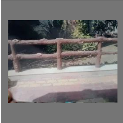
Artificial cement Wooden Pillars
