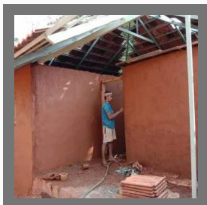
Mud House Construction Services
