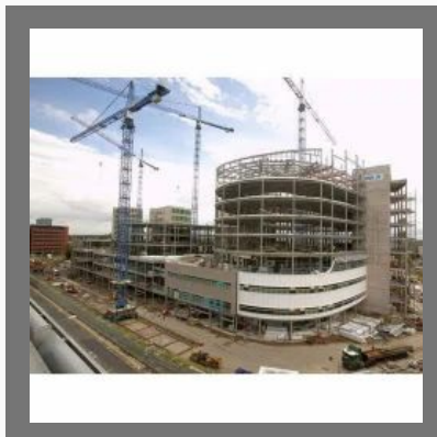
Hospital Construction Service
