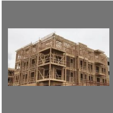
Apartment Construction Service
