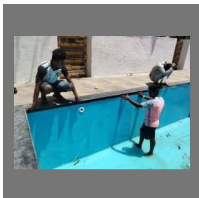
Swimming Pool Liner Installation Service
