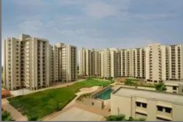
Apartment Buildings Construction
