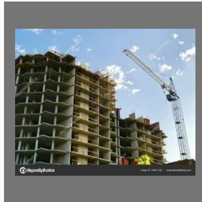
Appartment Building Construction
