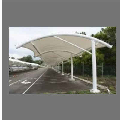
Car Parking Tensile Structure
