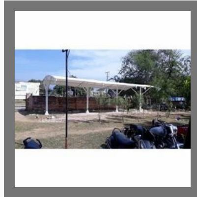
Car Parking Tensile Structure
