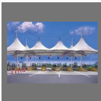
Toll Plaza Canopy Tensile Membrane Structure
