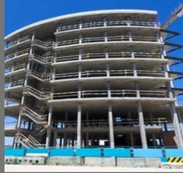
Structural Designing Services
