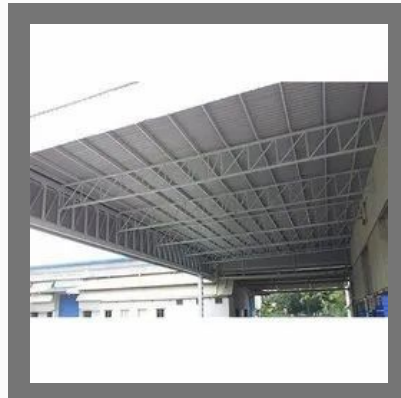
Industrial Roofing Sheet Fabrication Work
