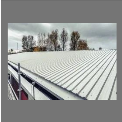
Industrial Sheet Metal Work
