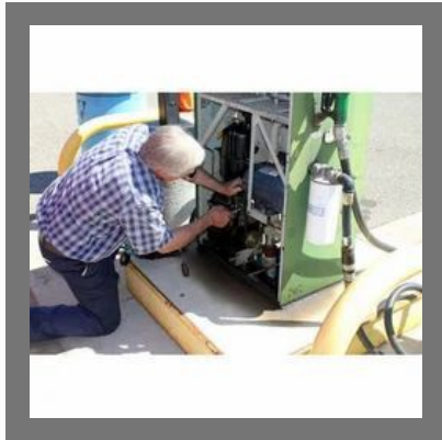
Fuel Dispenser Repairing Service
