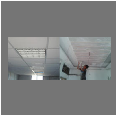
Gypsum Ceiling Service
