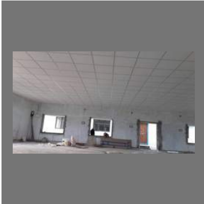
Thermocol False Ceilings
