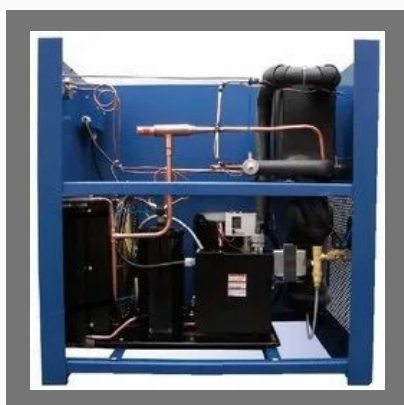
Compressed Air Dryer Repair
