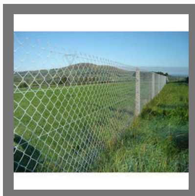
Chain Link Fence
