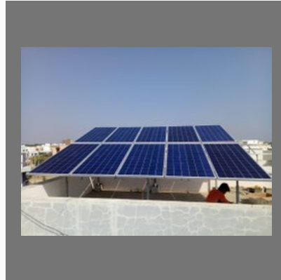
Commercial Solar Panel Installation Services
