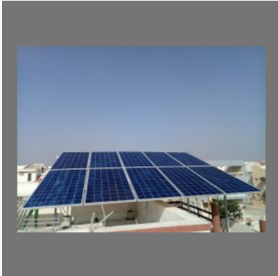
Residential Solar Rooftop Panels Installation Services
