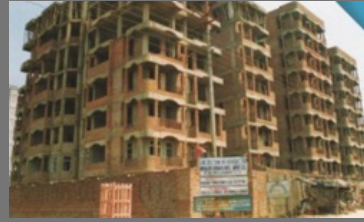
Construction of 120DU's Multi Storey (S + 8 ) Residential building
