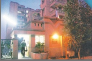
Construction of 72 DU's Multi Storey (S + 7) Residential Building
