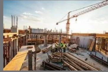
Commercial Building Construction Work
