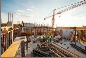
Construction Of Commercial Building
