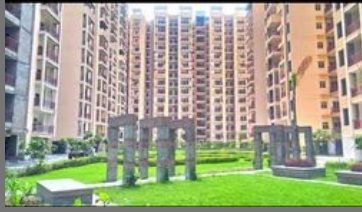
1 BHK Apartment Construction Service
