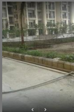
4 BHK Apartment Construction Service
