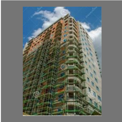
Multistory Building Construction
