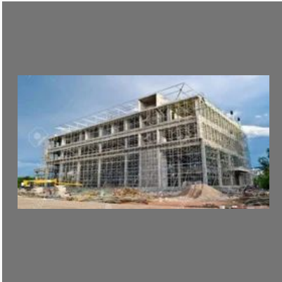
Mall Building Construction
