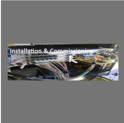
Installation & Commissioning Services
