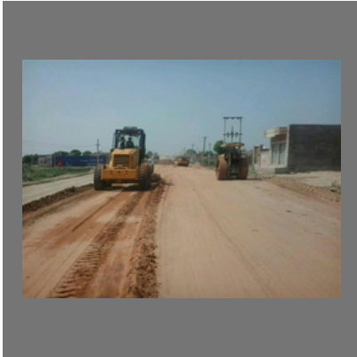
Roads Construction Service
