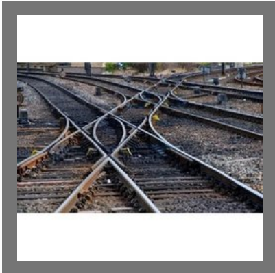
Railway Track Construction Service
