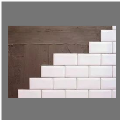
Wall Tile Fixing
