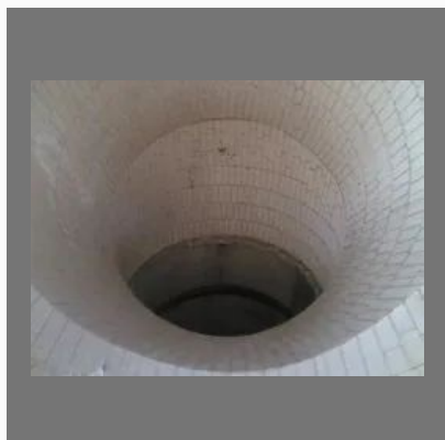
Refractory Lining Services
