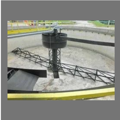
Clarifier With Scraper Mechanism
