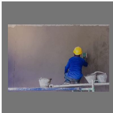
Wall Finishing Service
