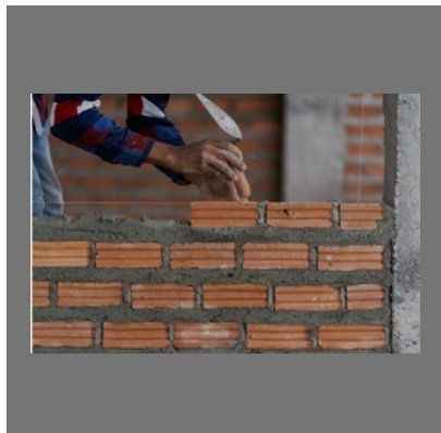
Basic Building Materials Service
