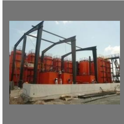
Electrical & Instrument Engineering
