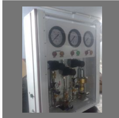
Oxygen Automatic Control Panel
