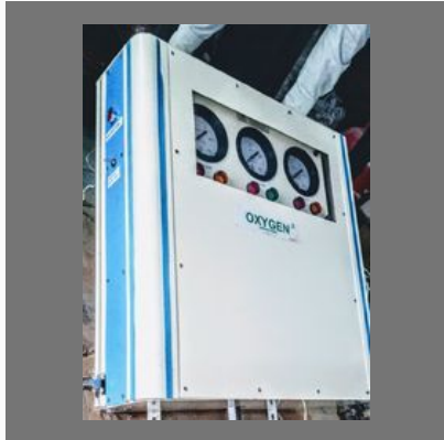
Oxygen Automatic Control Panel
