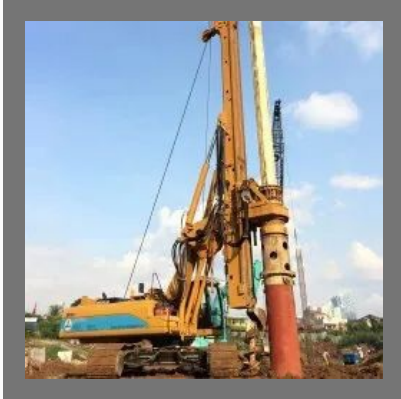
Borewell Drilling Services
