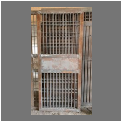
Iron Jali doors
