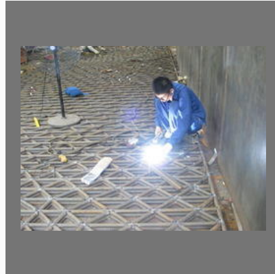
Steel Fabrication Work
