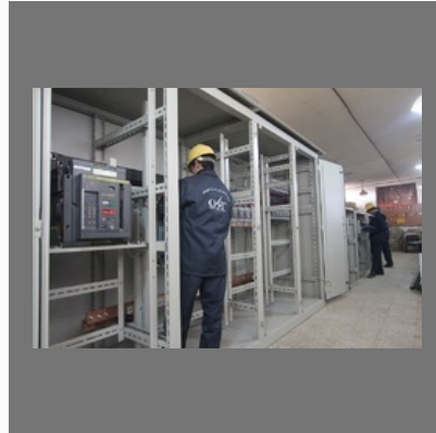
Panel Board Fabrication Work
