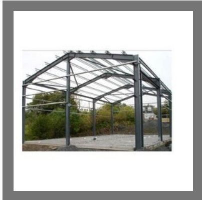
Shed Fabrication Work
