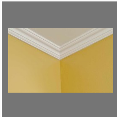
Gypsum Ceiling Cornice
