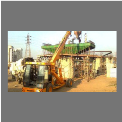
Repairs And Rehabilitaiton Of Structure Services
