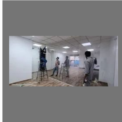
Office Glass Partition
