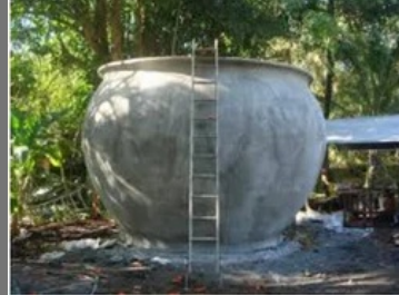
Water Tank Construction Service
