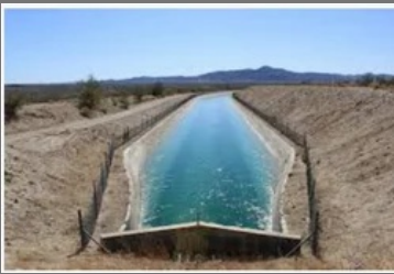
Aqueduct Construction Service
