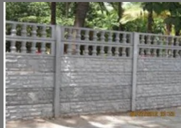
Compound Wall Construction Service
