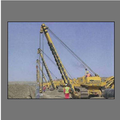
Pipe Lines Services
