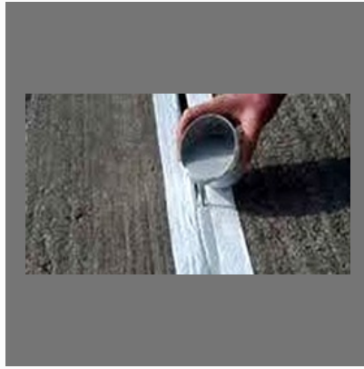
Polysulphide Sealant Service
