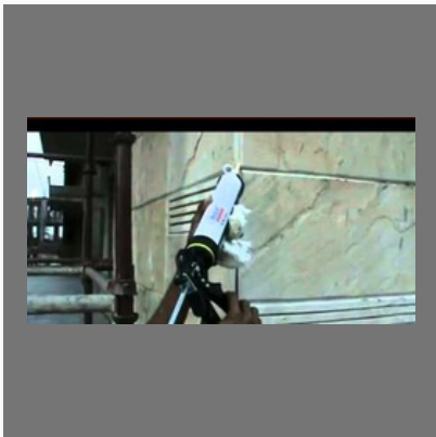
Polyurethane Sealant Service
