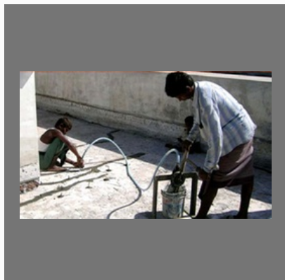
Pressure injection Grouting Service
