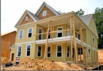
House Construction Services
