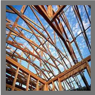
Ceiling Angle Frame Work
