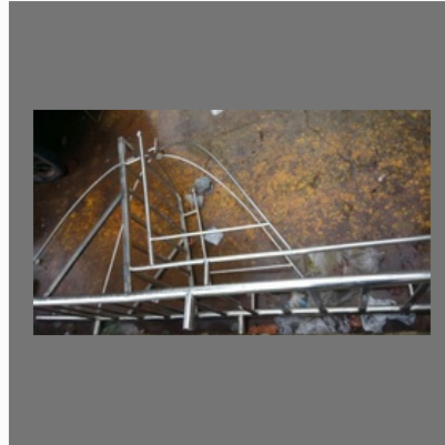
Steel Fabrication Work
